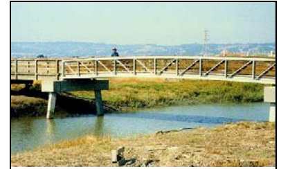
San Lorenzo Creek Bridge
