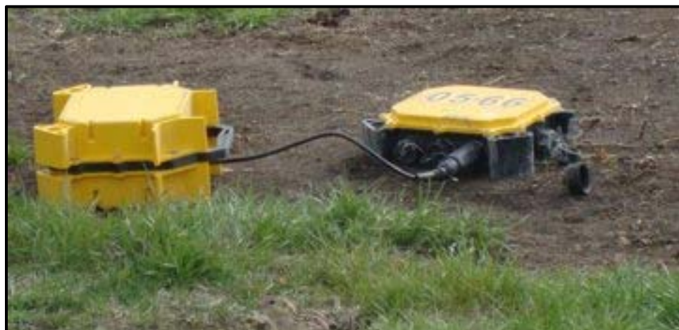
Figure 1-7b. Typical Wireless Iseis Sigma Nodal Land Recording System Installation (Battery Pack is located on the left and Recording System on Right)
