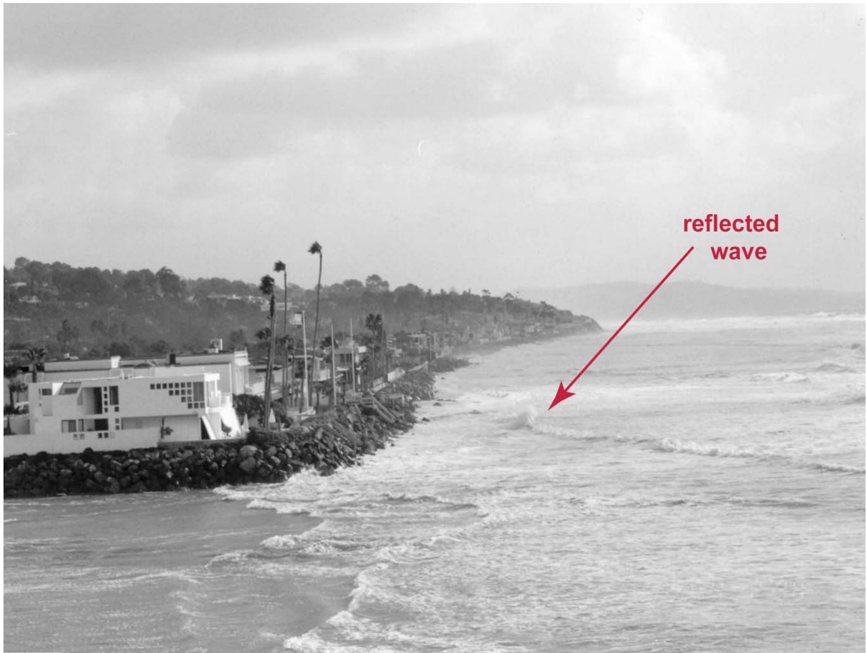
Figure 30. Reflected wave from Sandy Lane revetment (seawall) during winter erosion cycle - 4 February 1998.
