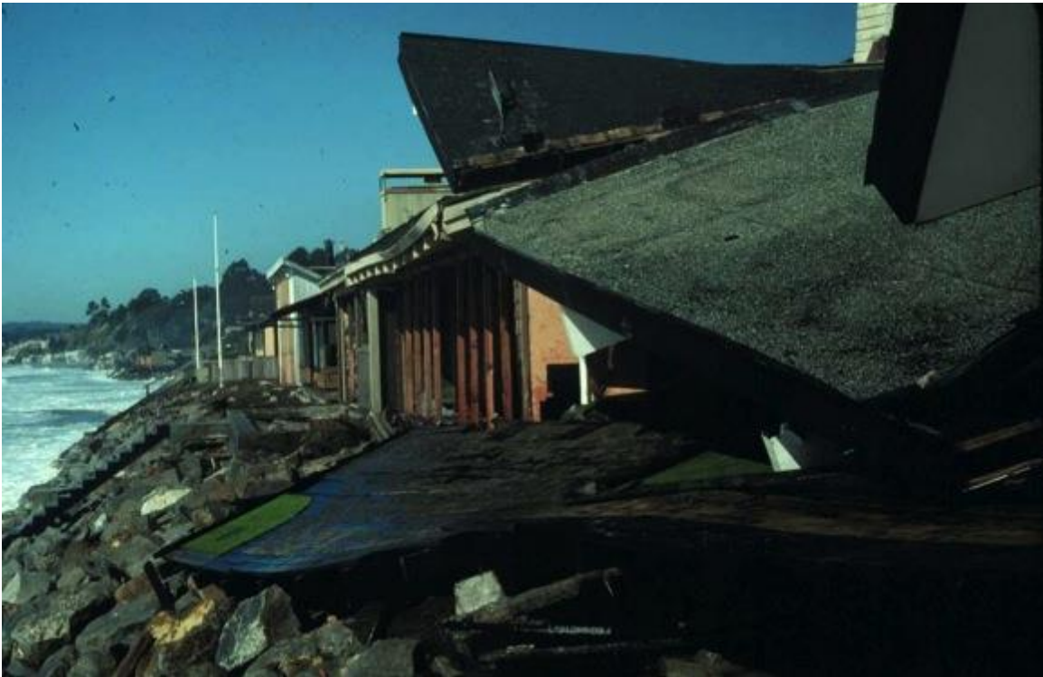
Via Gaviota, Aptos Seascape 1983 Damage from wave impact
