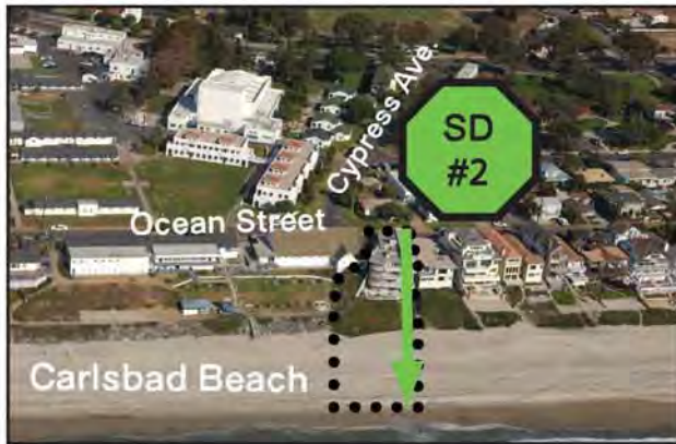
SD # 2 - Beach Access Stairway, 2601 Ocean Street, City of Carlsbad. OTD recorded 1983. Permit # A-77-81 for three condominium units.
