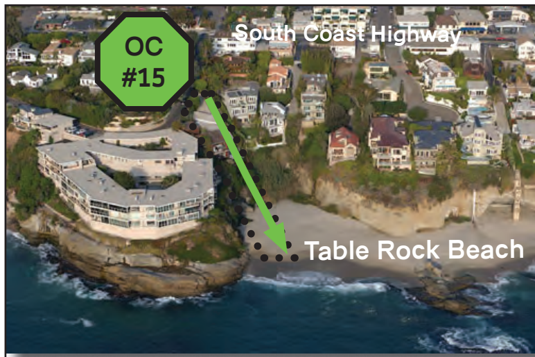
OC # 15 - Beach Access Stairway, 31625 South Coast Highway, City of Laguna Beach. OTD recorded 1984. Permit # 5-83-482 for one SFD and public stairway to beach.
